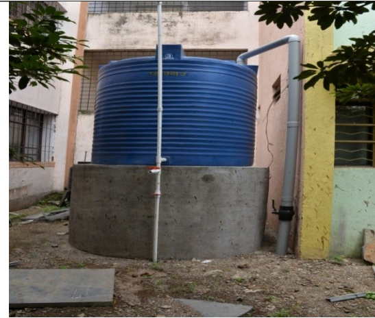
Rain Water Storage tank PG Building
